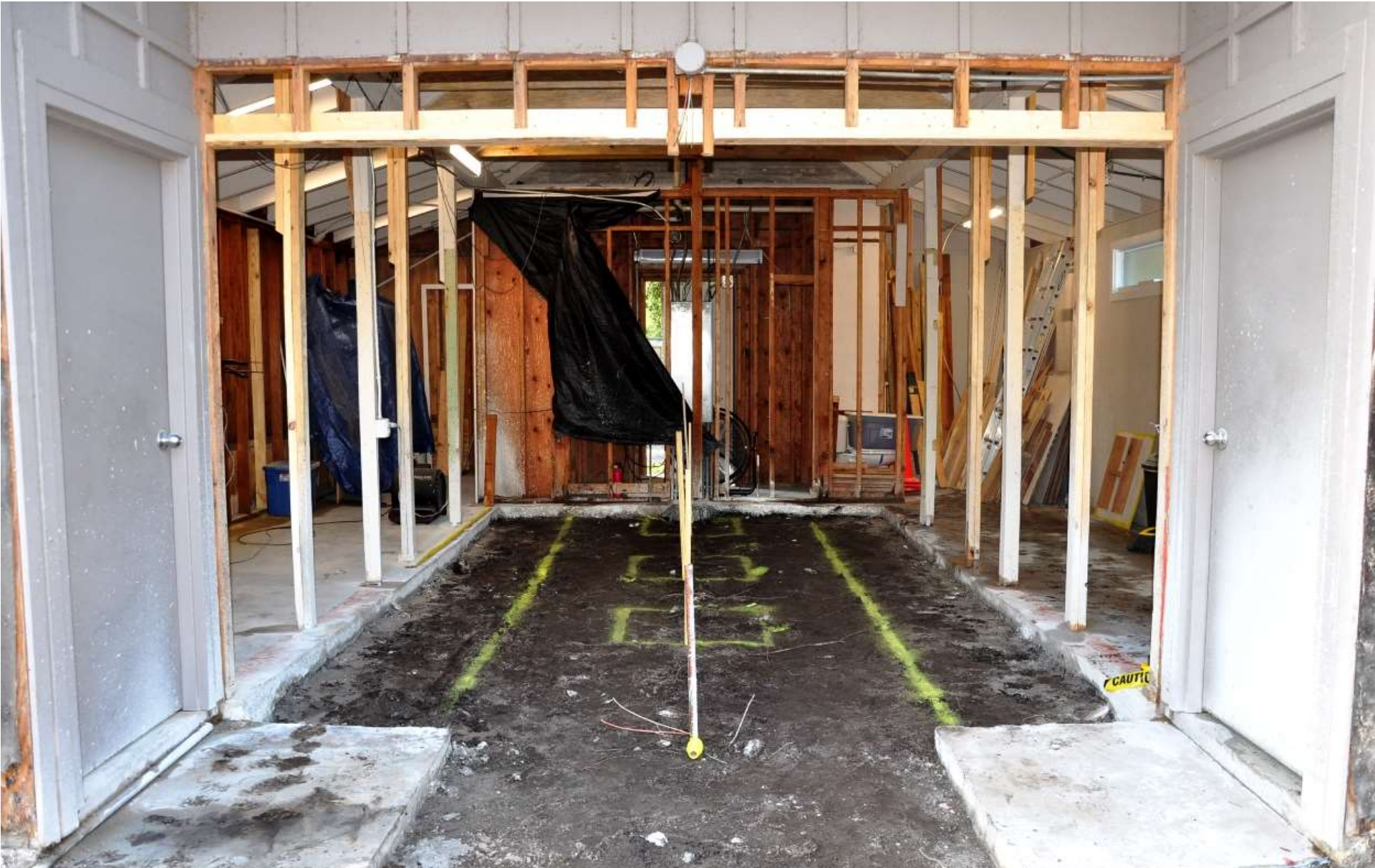
CENTER SLAB AND FRAMING REMOVED
