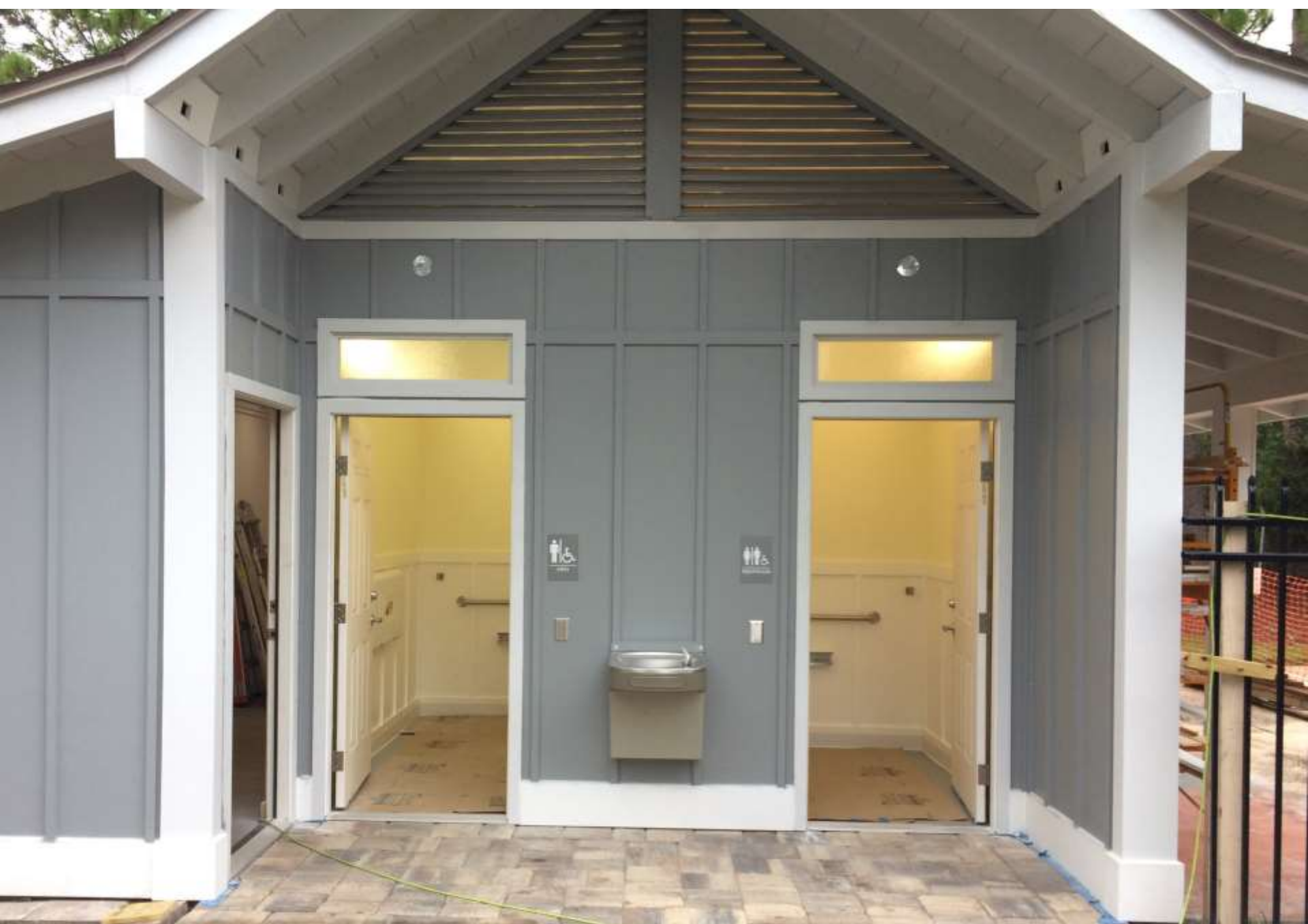
TWO NEW ADA-COMPLIANT RESTROOMS
